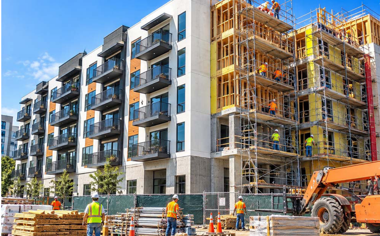
Construyen apartamentos en California, mientras votantes consideran bono de $11,250 millones para viviendas asequibles. Workers build apartments in California as voters consider an $11.25 billion affordable housing bond.
